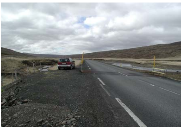
1 h3-05 Hringvegur, Fornihvammur
